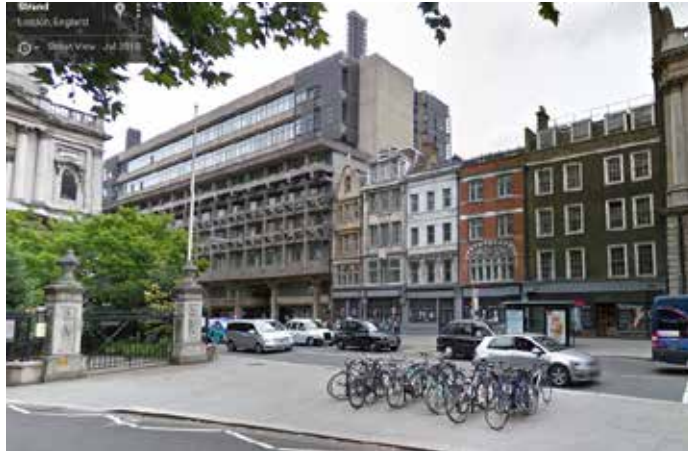
Nos. 152-158 The Strand as existing. Formerly known as the 'Old Law Building', this row of houses on their original narrow medieval plots encompass a wide range of styles, from a characteristic London stock brick façade, to a playful re-rendering of a Georgian house, to Arts and Crafts flamboyance and early 20th-century interpretations of the Dutch style. To the left is the Brutalist building.
