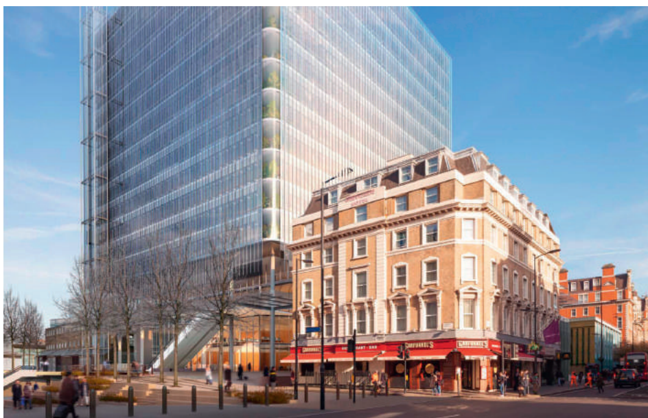
The site with the Edwardian sorting office (top) and the proposed development (bottom) (Image: planning application documentation)
