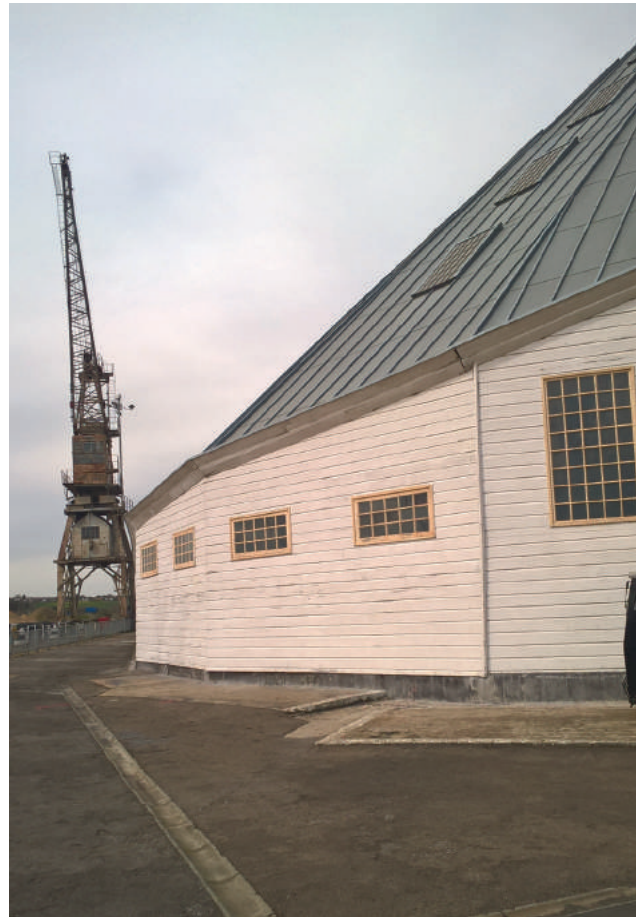
No. 3 slip from the outside
