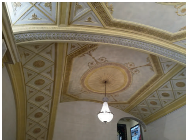
The historic ceiling in the foyer
