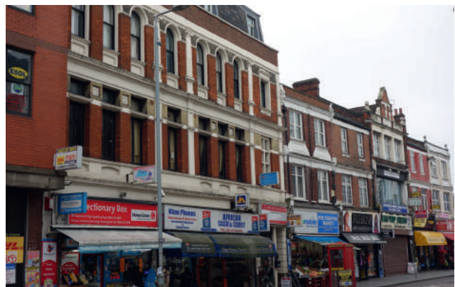
The site seen from the west
