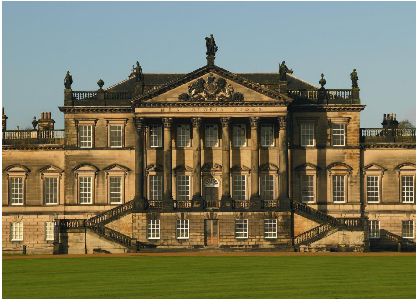
The east front of Wentworth Woodhouse, where negotiations over the acquisition of the house continue. Country Life
