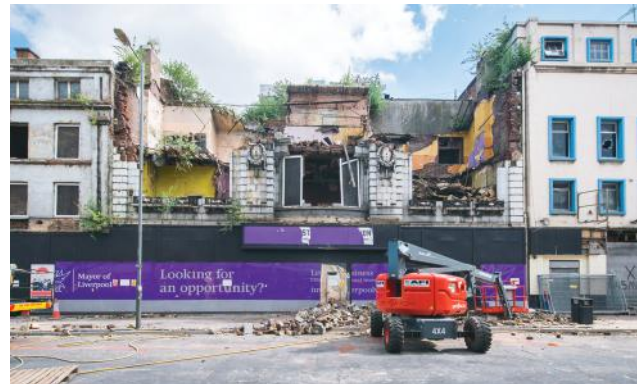
The Futurist Cinema, during demolition. http://johnjohnson-photography.com
